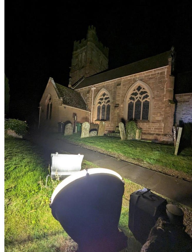
Figure 15 - How not to illuminate. Inappropriate luminaires used to illuminate a heritage asset with significant landscape impact (not in Oxfordshire). Credit Dan Oakley
