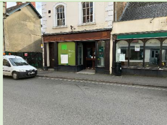
Figure 4: The vacant former Budgens unit on Marlborough Street. Stakeholders referenced the role that out-of-centre operators, such as Tesco, have played in reducing the performance and role of the town centre in meeting shopping needs.
