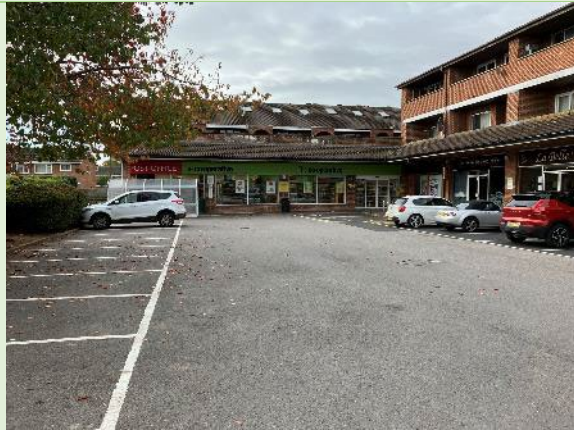
Figure 1: Grovelands Shopping Centre is enclosed and lacks significant levels of either natural or passive surveillance. The Centre is anchored by a Co-op Food, which clearly drives activity into this location and supports any linked trips that occur.
