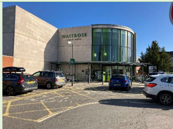
Figure 4: The Waitrose foodstore on St Martin’s Street underpins the convenience goods offer in Wallingford and clearly drives a significant level of pedestrian footfall in the town.
