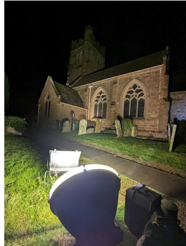
Figure 15 - How not to illuminate. Inappropriate luminaires used to illuminate a heritage asset with significant landscape impact (not in Oxfordshire). Credit Dan Oakley
