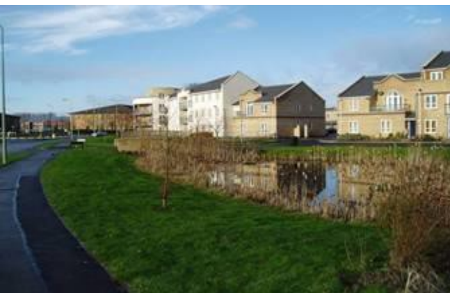
Figure 7 Example of a retention pond.
