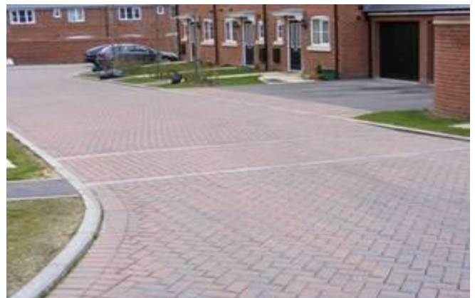
Figure 10 An example of permeable paving.
