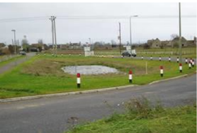
Figure 8 Example of a detention basin.
