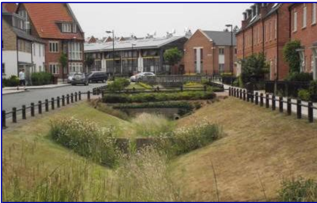
Figure 6 An example of a swale.
