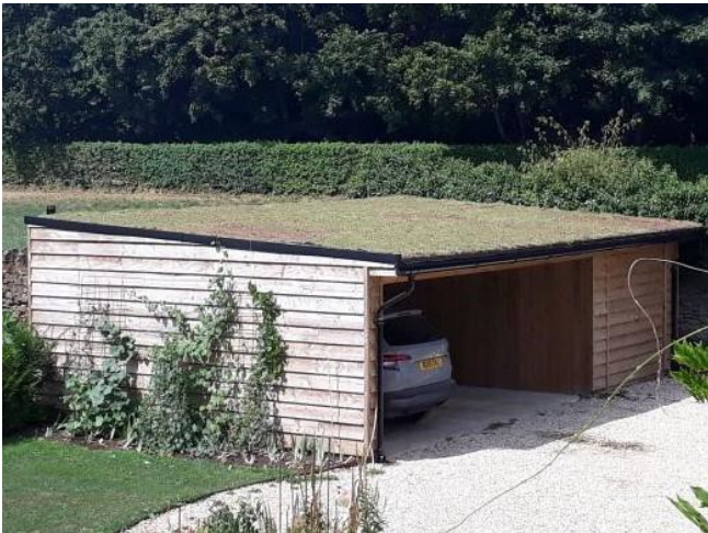
Figure 1 An example of a sedum green roof (photo: © Oxford Green Roofs Ltd)
