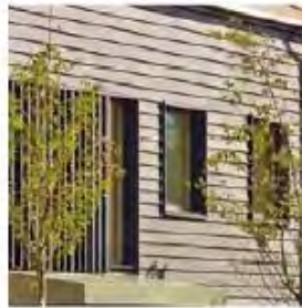
Horizontal wood cladding
