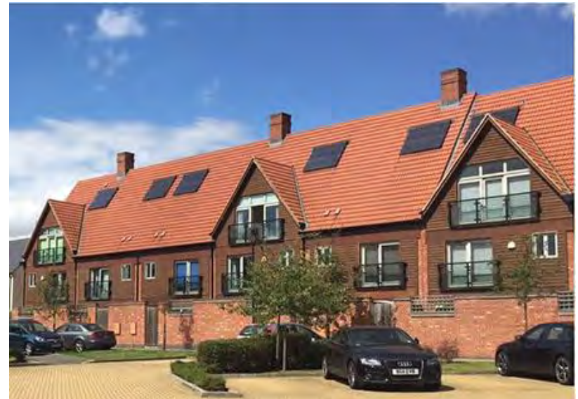
Example of an attractive rear courtyard with integrated planting and natural surveillance (Upton, Northamptonshire)
