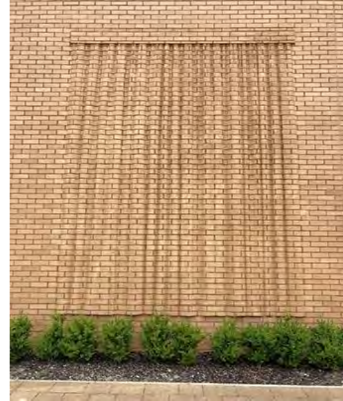
Brick relief, district centre wall (Didcot)
