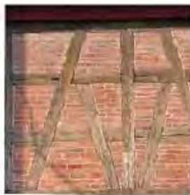
Light framing (studs) with brick
