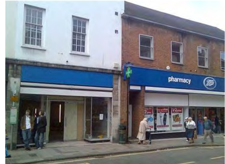
3 Bell Street, Henley before refurbishment
