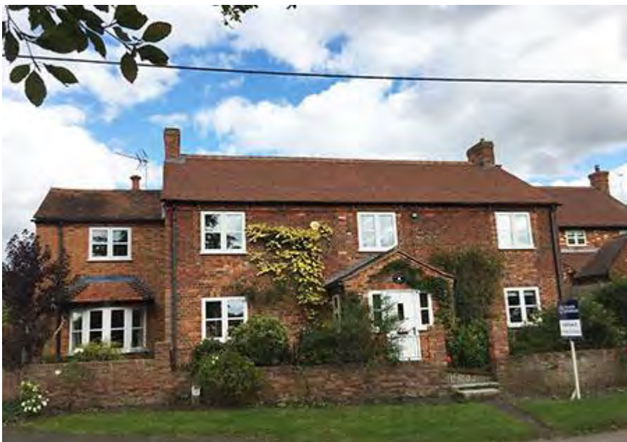
Extension in keeping with the existing character and appearance of the house (Kingston Blount)
