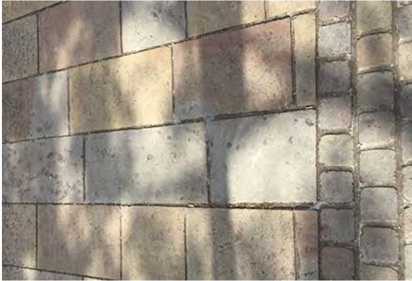
Hard wearing and long-lasting buff block paving (Thame)
