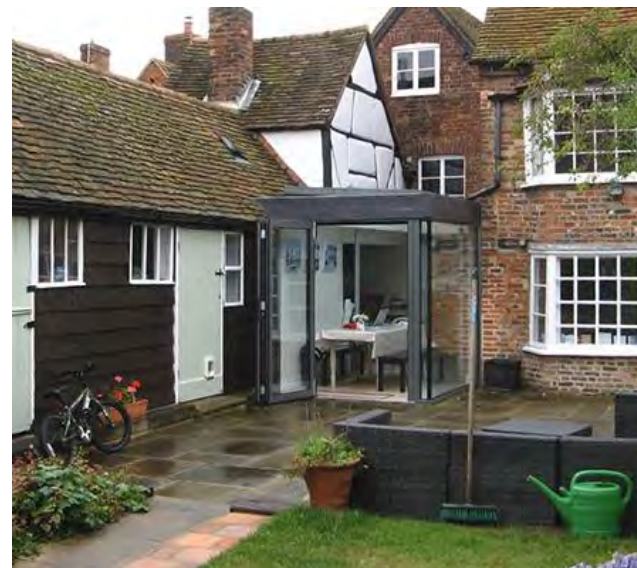
Successful contemporary extensions to a traditional building in Watlington
