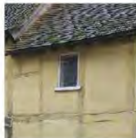
Light framing (studs) with render
