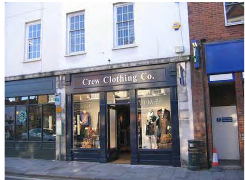
3 Bell Street, Henley after refurbishment
