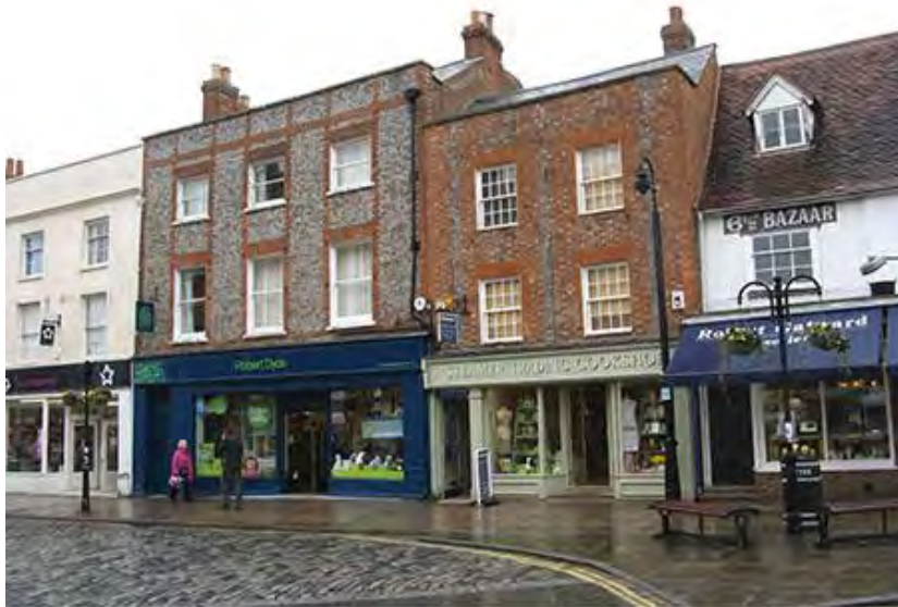
Example of traditional shopfronts along a street (Thame)
