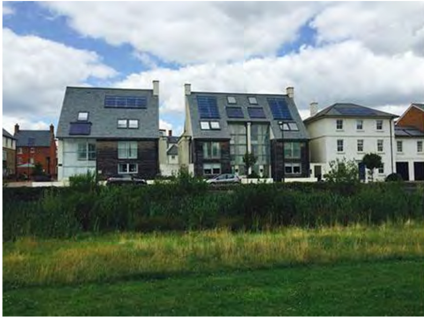
Photovoltaics (Upton, Northamptonshire)
