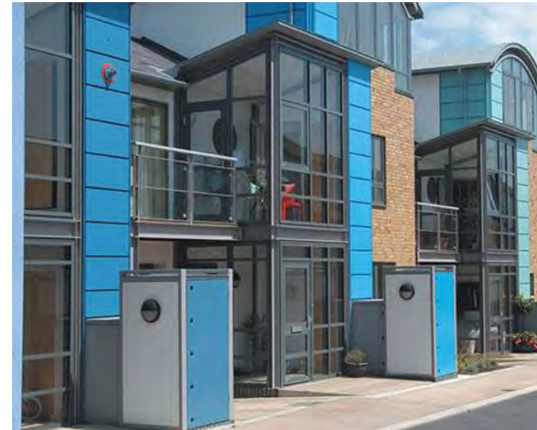
Bin storage areas should be considered as part of the architecture (Newhall, Harlow)
