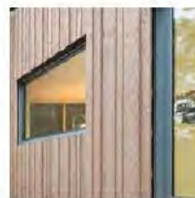
Vertical wood cladding
