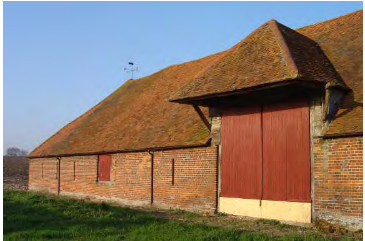
Should any conversion take place at sites like this it would be important to retain the integrity of the roofs and walls. (Ipsden)
