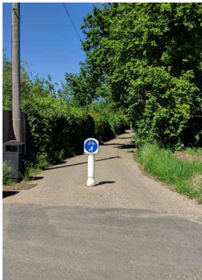
Placement of a single bollard to prevent vehicles from entering the cycle path
