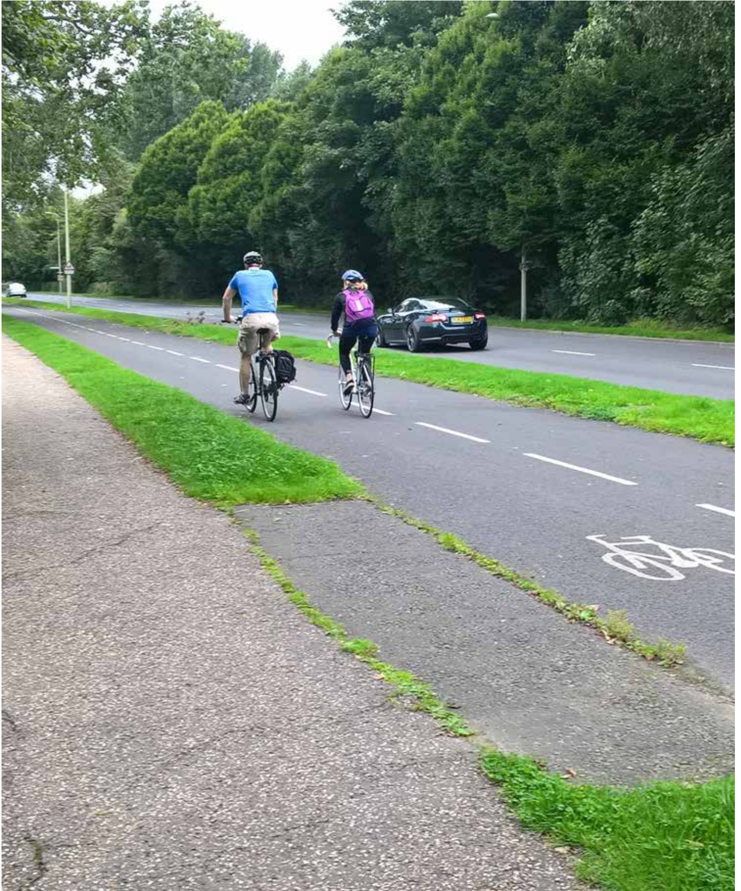
Marston Ferry Road, Oxford. Cycle users have a wide track (centre of photo), pedestrians have a separate track separated from the cycle path with a verge (left of photo), motor vehicles are separated from both (right of photo)
