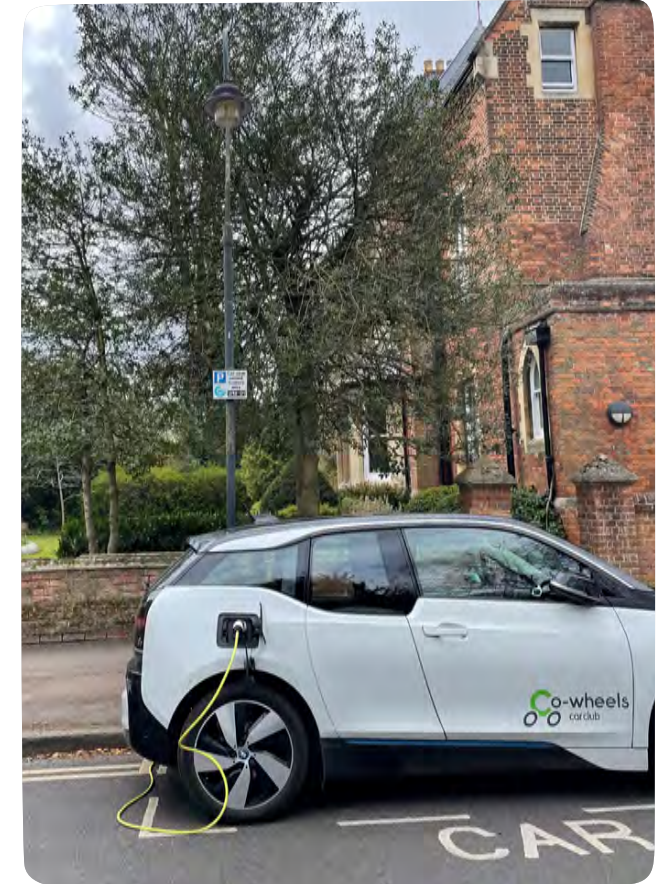
Electric vehicle charging point.
