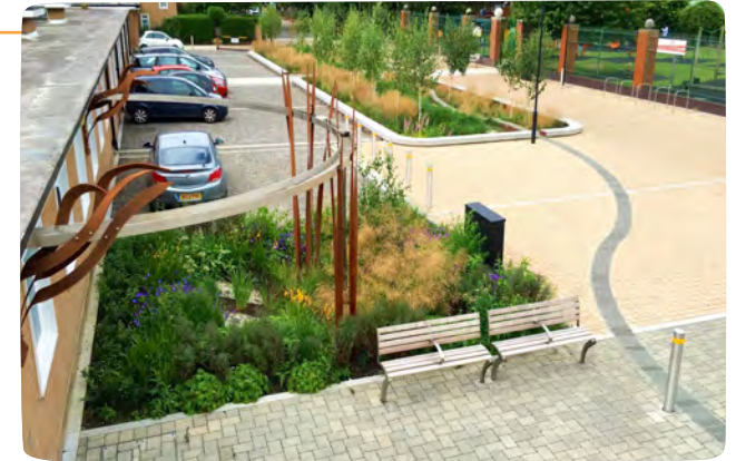
Rain gardens in the public realm: Non adoptable if taking water from private areas.
