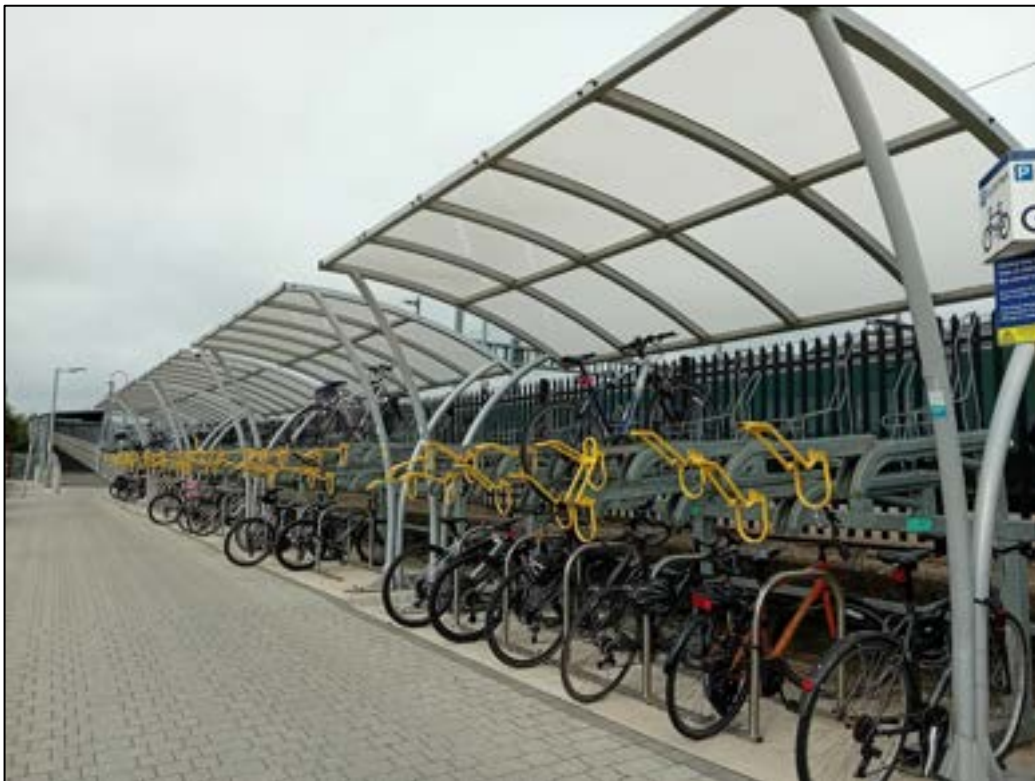
Figure 18: Covered 2 tier stands at Didcot Parkway Rail Station, Didcot
