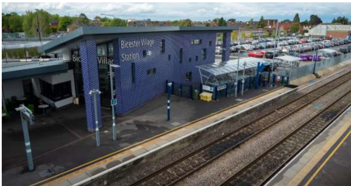
Figure 27 – Photo of Bicester Village Station which was delivered during Phase 1 of East West Rail
