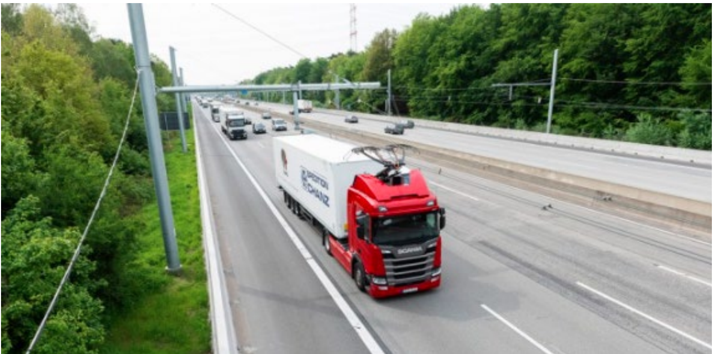
Figure 10 – Electrified road system trial 45
