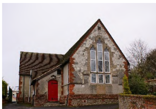
Figure 7.11: Grade II Former School, now village hall
