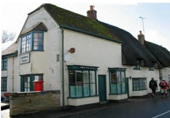
Figure 3.9: Former Post Office - this facility has now been accommodated part-time in the Rose and Crown
