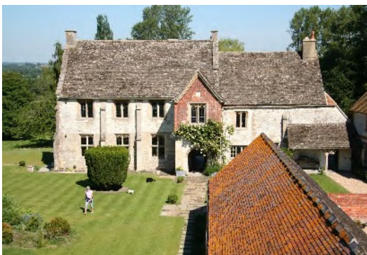
Figure 7.10: Grade II Manor House
