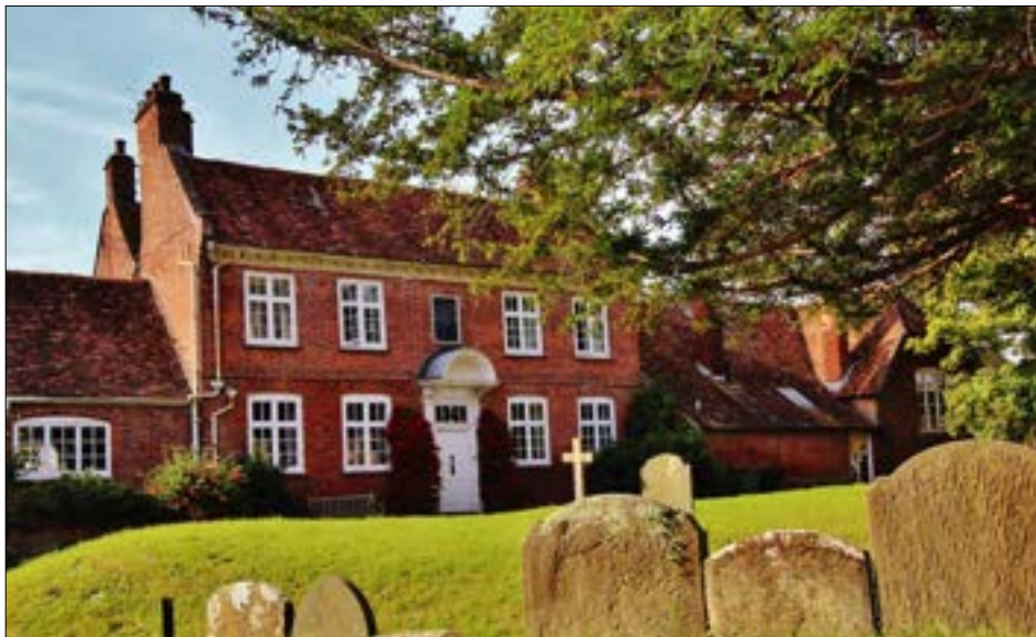
Figure 46: The Old Schoolhouse, viewed from the Churchyard.
