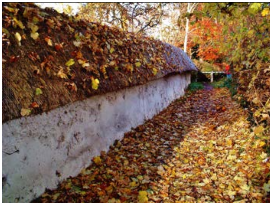
Figure 8: Thatched cob wall
