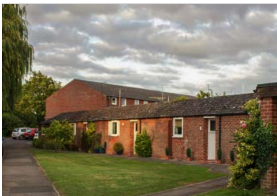
Figure 26: Single-storey housing for over-55s at Dibleys
