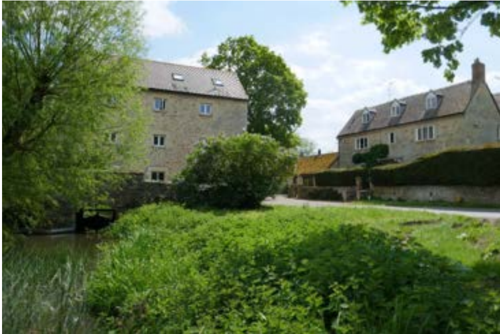
Figure 3 Heritage Group A Cuddesdon Mill and Mill House
