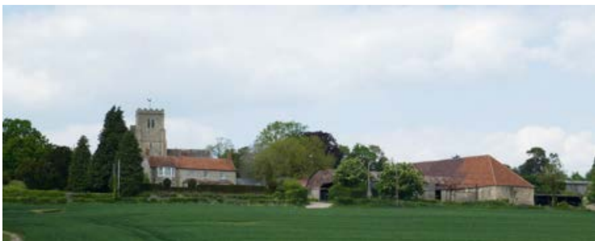
Figure 4 – Part of Heritage Group B: Dove House and Dove House Farm Barn
