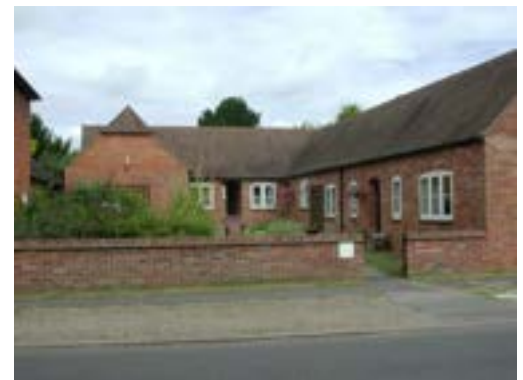
Alms Houses, High Street, Drayton
