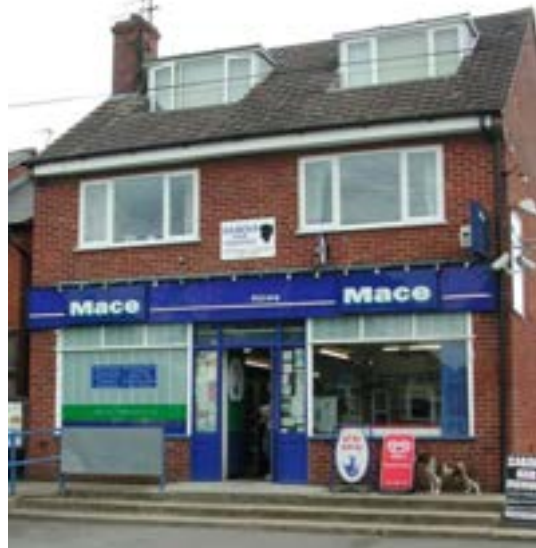
Mace Shop, Abingdon Road, Drayton
