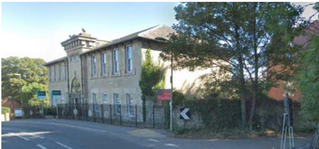
Figure 14. The former Nalder manufacturing works (now residential properties), an example of limestone construction.
