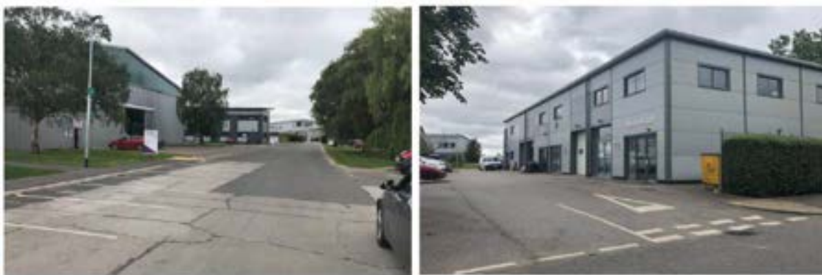
Figure 45. Grove Business Park
