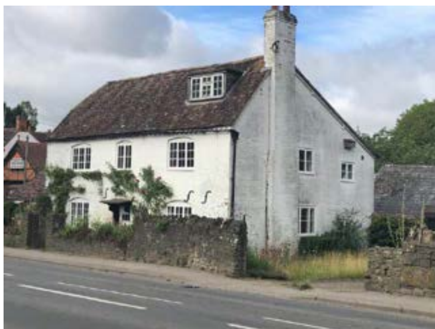
Figure 42. Listed building. Bridge House, 17 th century, remodelled in 18 th century
