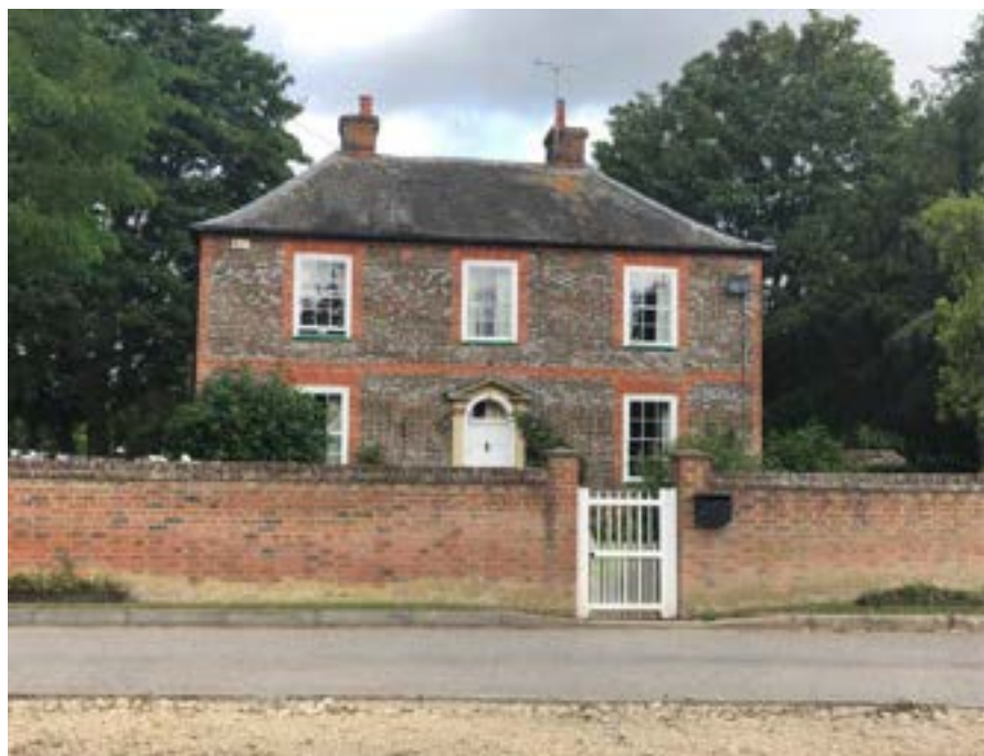
Figure 37. Listed building 18 th century farmhouse.
