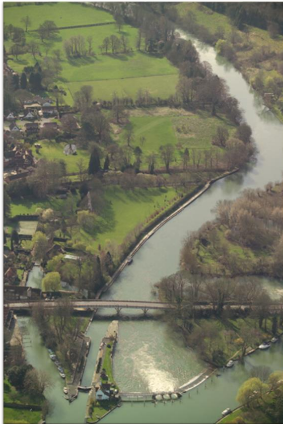
Figure 53 Goring weir and southwest floodplain
