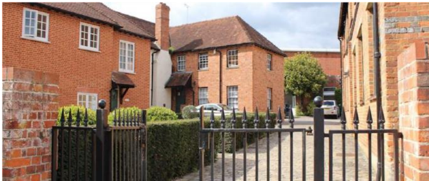
Figure 84 Thames Court business units, the High Street
