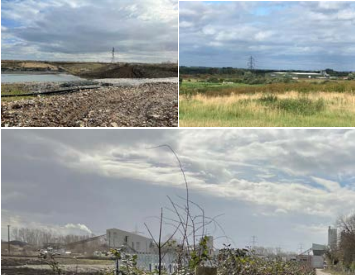
Figure 9.19, 20 & 21. Views of Operational Landfill & Composting Facility
