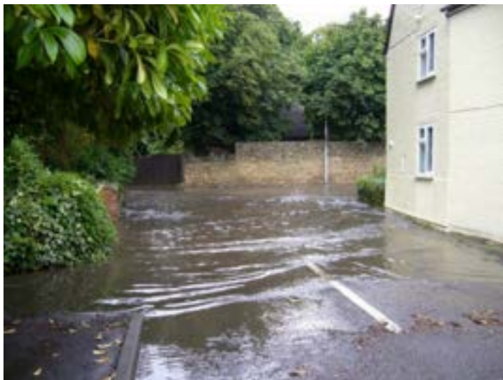
Figure 7.4 Brook Street/Chapel Lane Flooding
