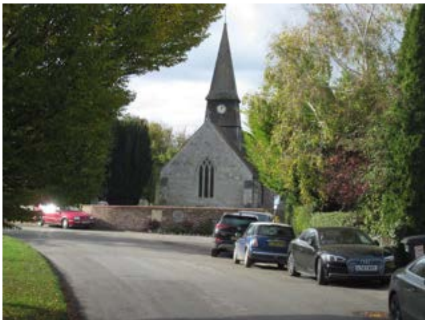
View of St Mary's from village green
