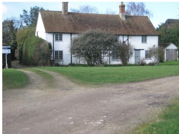
Timber-framed brick & render & tiled house
