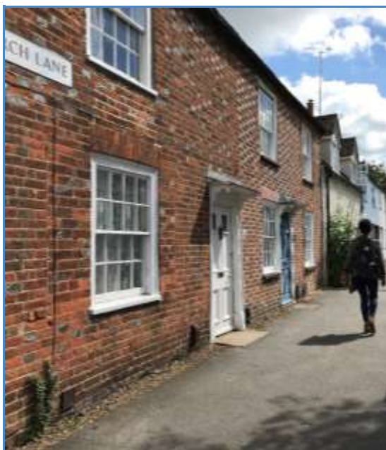
C18 vitrified header brickwork, Church Lane
