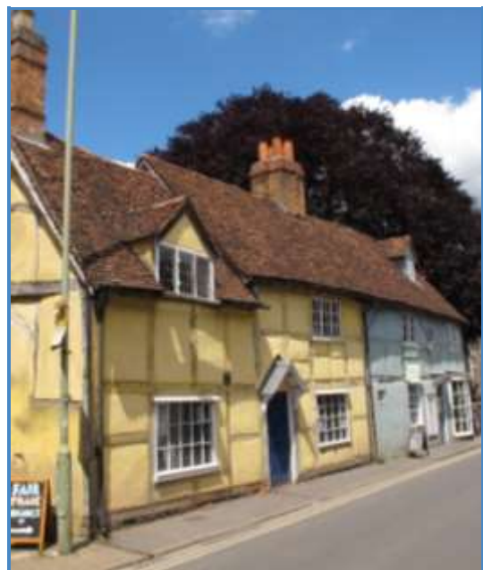
Timber framing, St. Mary's Street
