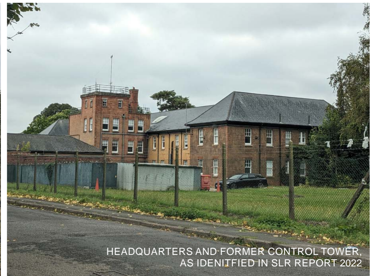
VIEW OF THE SITE LOOKING EAST FROM GOZZARDS FORD
