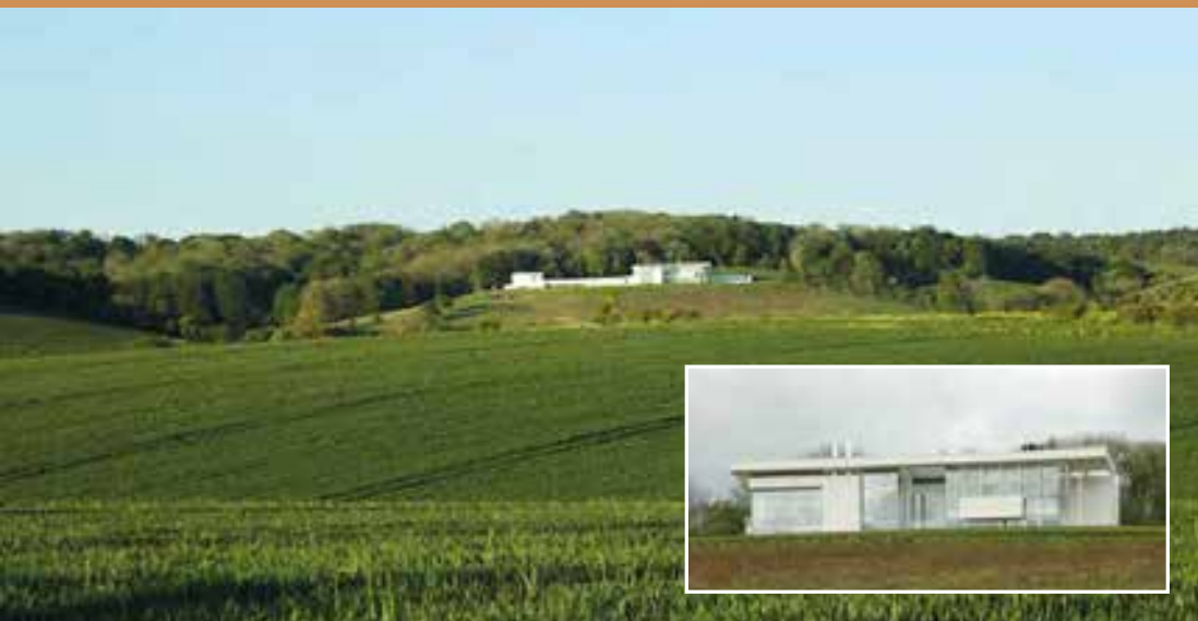
Grand new build projects can also be insensitive to the AONB. Stark, white, huge and angular this replacement dwelling, here viewed from the Chilterns cycleway, dominates the landscape in its siting and design.
