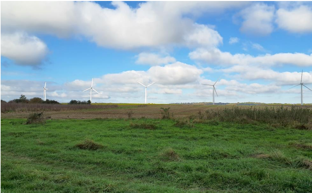
Figure A.24: Westmill Wind Farm near Watchfield
