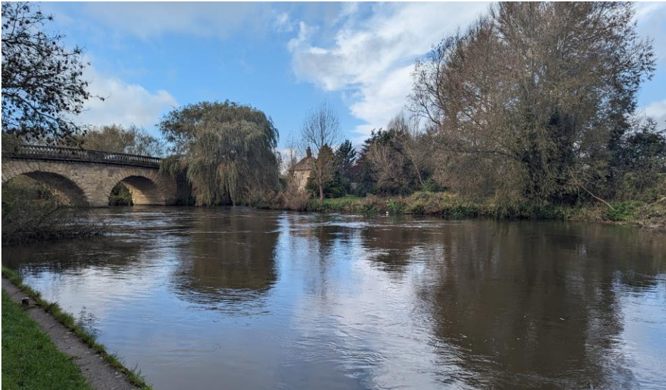
Figure A.38: Swinford toll bridge
