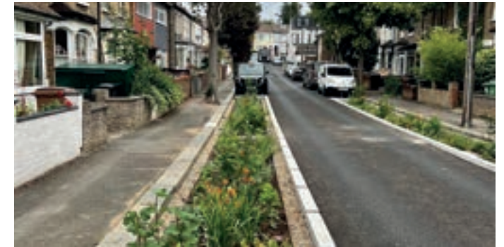
Street rain gardens © Meristem
