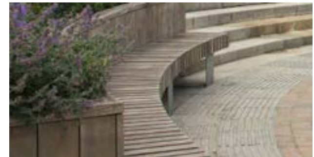
Pocket Park Areas: Extensive raised planters with timber edge seating (example: Orchard Centre)
