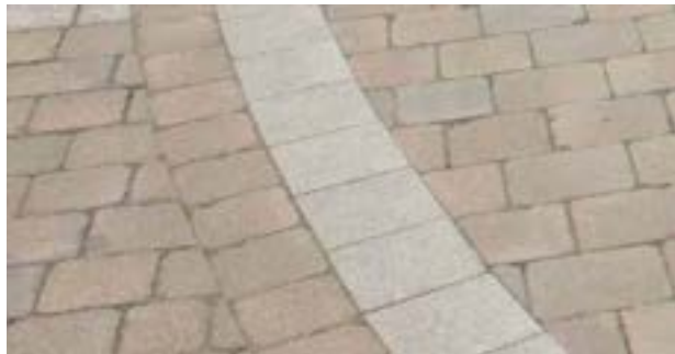
Public Realm Areas with Traffic: Red brick setts with flush concrete kerbs - as used within the Station Road-Broadway junction area
