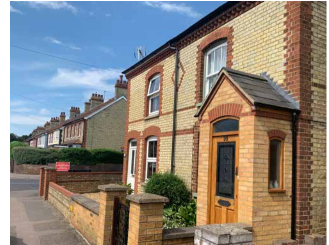
Figure 55: Positive example of a front extension.
