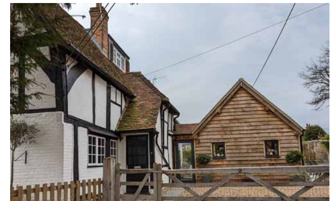
Figure 57: Local positive example of a side extension that respects the existing building in terms of scale and building materials. In particular, the use of weatherboarding positively reflects back to the typical appearance of barns and outbuildings.
