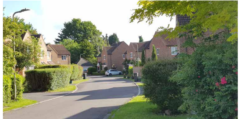
Figure 21: The roofline along Bishops Orchard is generally regular, whilst the roof types range between gabled and cross gabled roofs.
