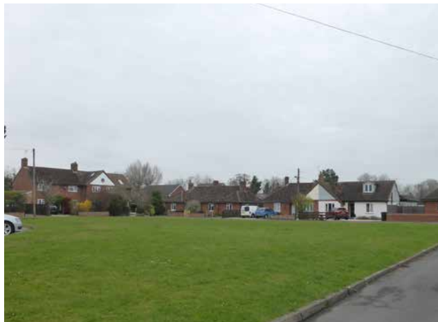
Figure 30: The open space along Windsor Crescent offers a feeling of openness in the area, whilst as properties overlook the open space, the natural surveillance is enhanced.
