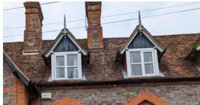
Gabled dormer with brick chimney
