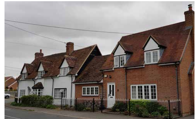
Figure 44: Any new development in close proximity to listed buildings should sit sensitively next to them respecting its scale and massing whilst allowing for a green buffer in between to mitigate visual impact.
