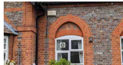
Varied brickwork with attractive detailing
