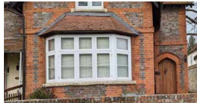
Bow window with hipped roof
