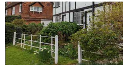
Stretch of painted metal railing
