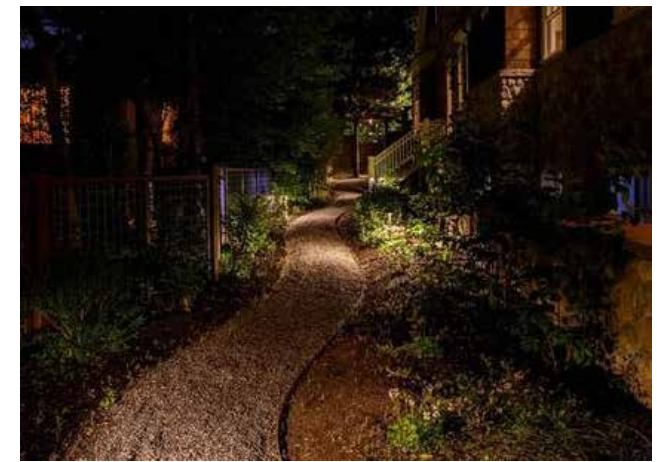
Figure 68: Example of path lighting where all lights are directed downwards, whilst the light sources are obscured.
