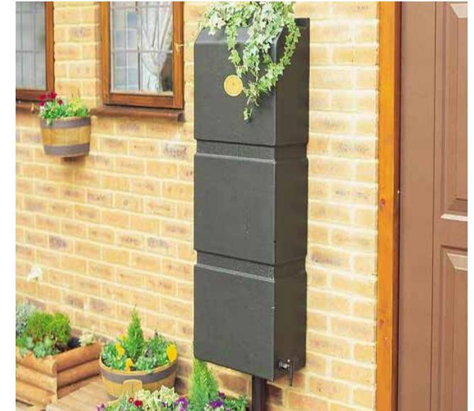
Figure 87: Example of a gravity fed rainwater system for flushing a downstairs toilet or for irrigation.
