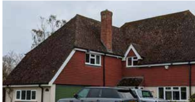
Half-hipped roof with clay tiles
