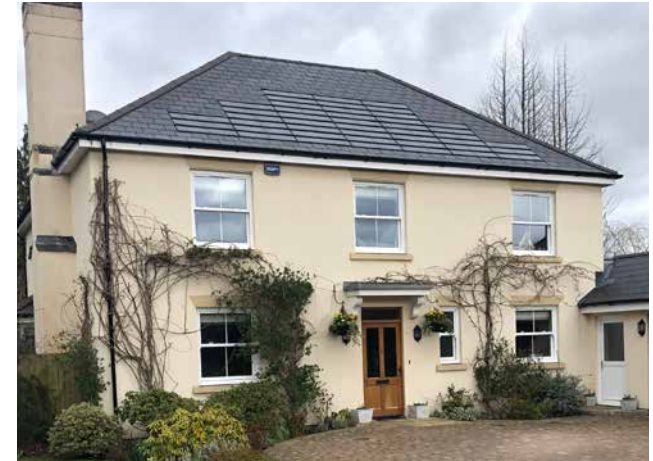
Figure 94: Use of shingle-like solar panels on a slate roof, with the design and colour of the solar panels matching those of the adjacent slate tiles.
