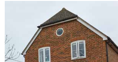
Dutch roof with clay tiles
