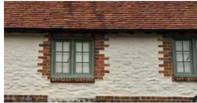
Rendered brick with red brick around the window frames
