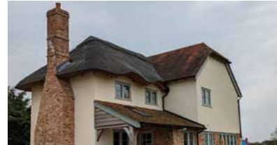
Thatched roof attached to a mansard roof and a brick chimney on a new home in East Hagbourne
