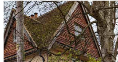
Tile hanging applied to decorative gable ends
