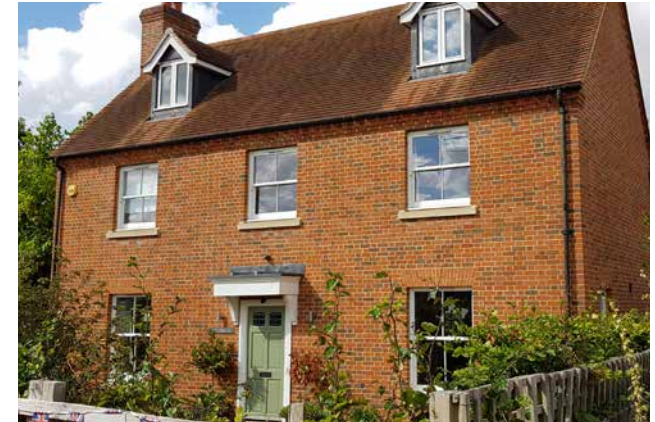
Figure 50: Local example of 2.5-storey building where the roofline is interrupted with a brick chimney and gabled dormers.
