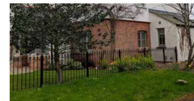
Metal railing & trees
