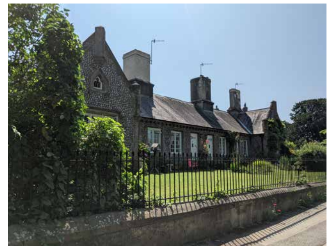
Figure 40: Positive example of a recent infill development (photo above) in a rural village elsewhere in UK that fits nicely into the local context (photo below) in terms of scale, massing, architectural styles and details.
