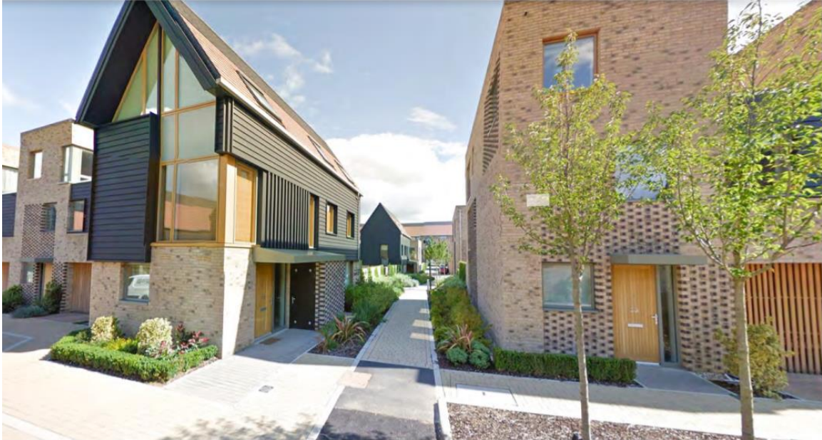
Figure 35: An example of a new development in Cambridge which was able to successfully incorporate alleyways, making them safe and attractive for use at all times of day, encouraging people to walk and promoting active and healthy lifestyles (image source: Google StreetView).
