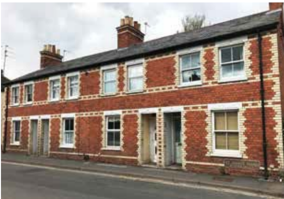
St John's Road first Municipal housing
