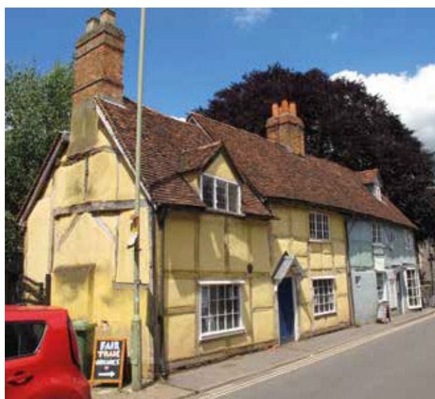
Timber framing, St Mary's Street
