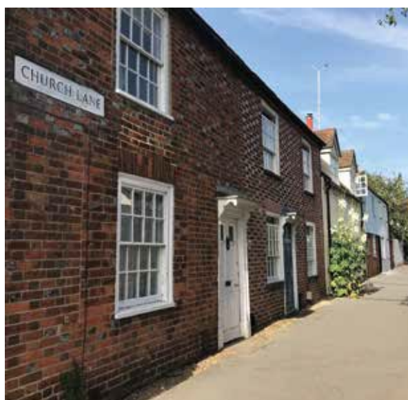
C18 vitrified header brickwork, Church Lane
