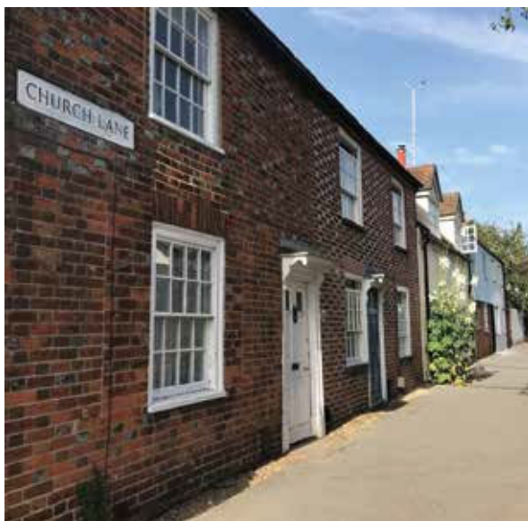
C18 vitrified header brickwork, Church Lane
