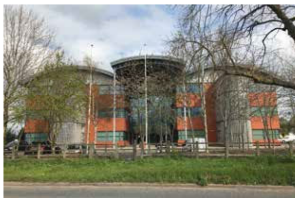
Former Habitat showroom and warehouse
