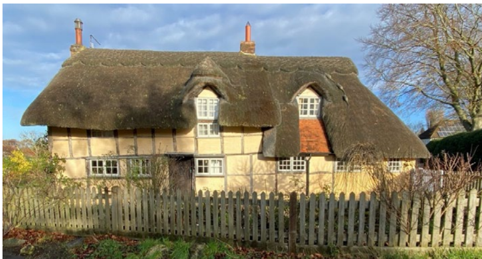
Fig 6. Thatch on The Stocks, possibly the earliest house in the village as it has a base cruck truss
