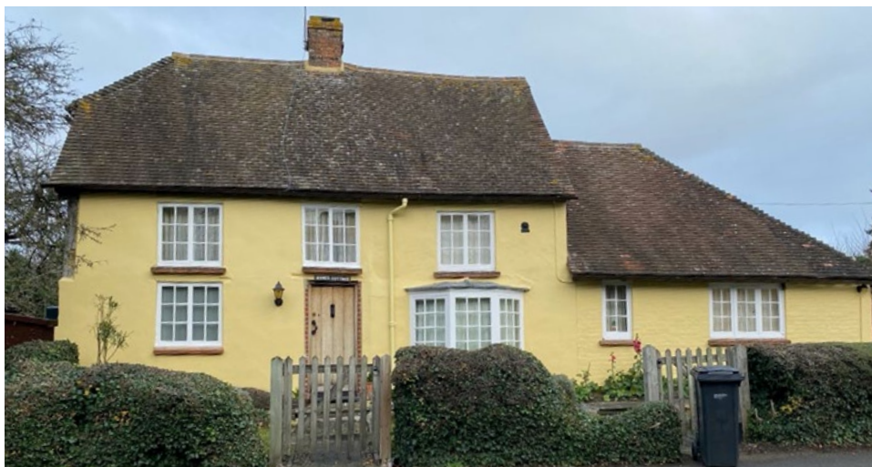
Fig 8. Ayres Cottage, London Road, showing a central stack in line with a central entrance, indicating a lobby entry plan
