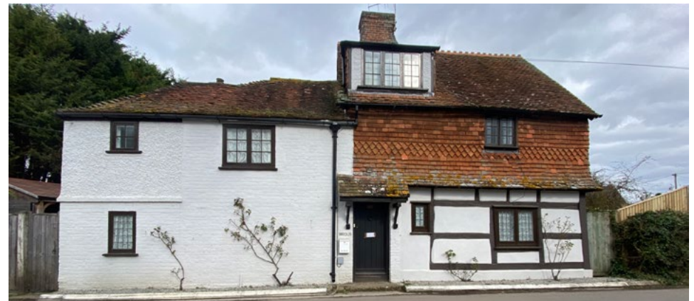
Bridus House, South Street
