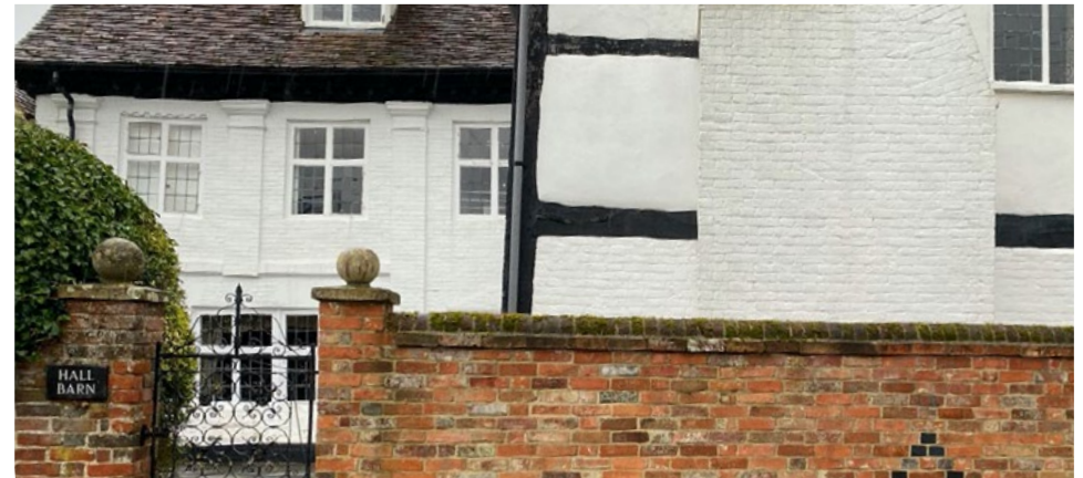
Fig 23. Hall Barn showing Doric pilaster in brick. Also visible is the external stack of the earlier timber-framed wing
