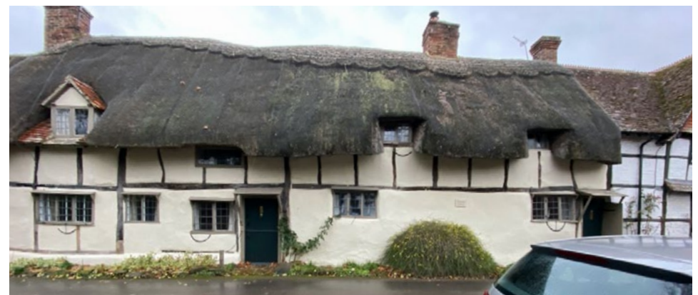
Fig 25. Wayside, late 16th century timber-framed house with thatched roof and inserted dormer
