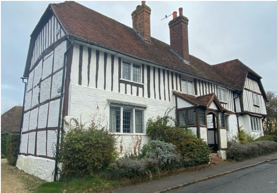
Fig 3. Close studding on the front elevation and upper gable of Corrydon House. The less visually prominent gable is constructed on the less impressive small square panels
