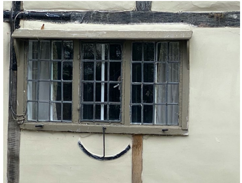
Fig 20. Early side-hung casement window, Wayside, Westbrook Street
