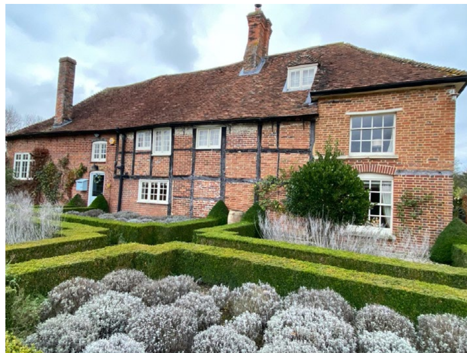
Fig 31. The Manor House, showing various phases of development, set in attractive gardens
