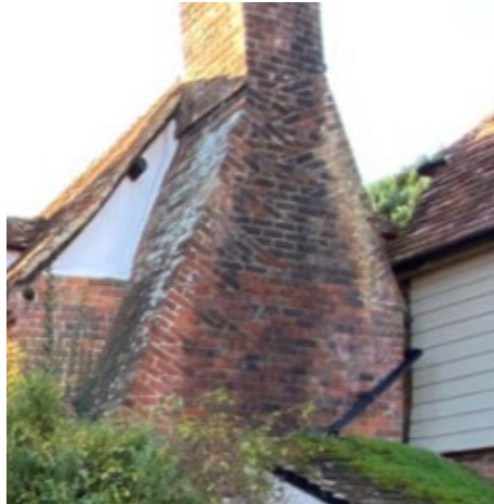
Fig 21. Chimney stack at Cherry Patch
