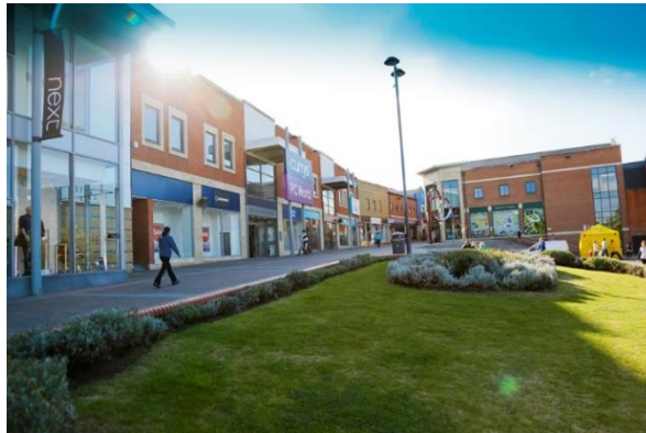
Figure 3: Didcot Town Centre
